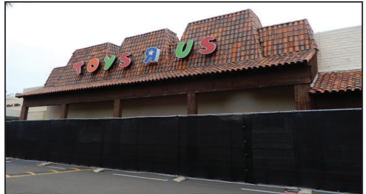
Burlington Coat Factory coming soon to 2425 Vista Way in the El Camino North shopping center.
